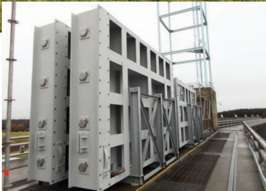
FIG. 5: Finished intake pieces were moved to a laydown area before being placed back in the water.
