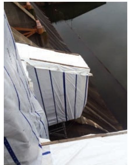
FIG. 7: Containment and scaffolding structures were constructed around tainter gates during the project.
