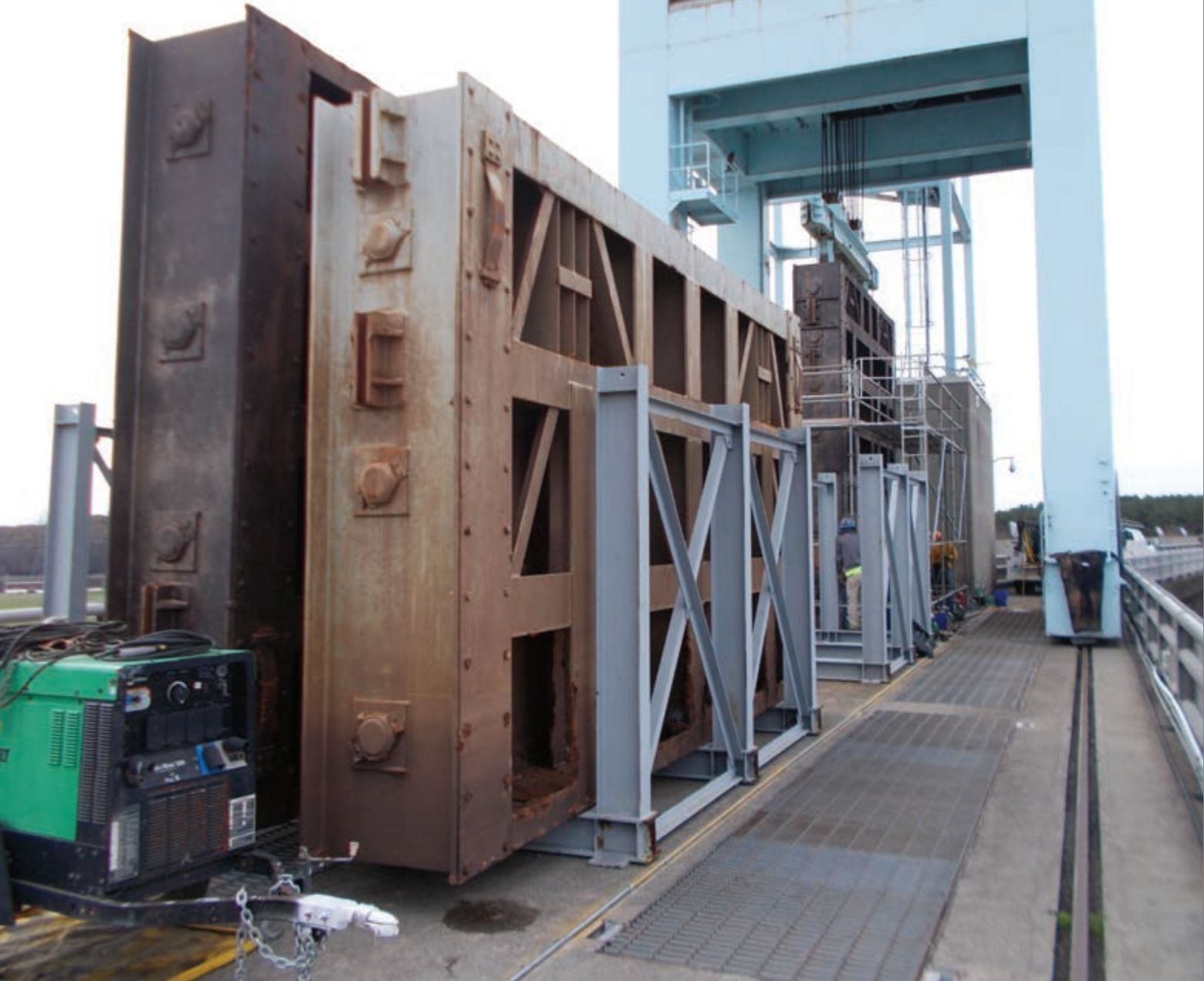
FIG. 2: Intake pieces were disassembled before being transported by crane to an onsite building for repairs, blasting and coating.
