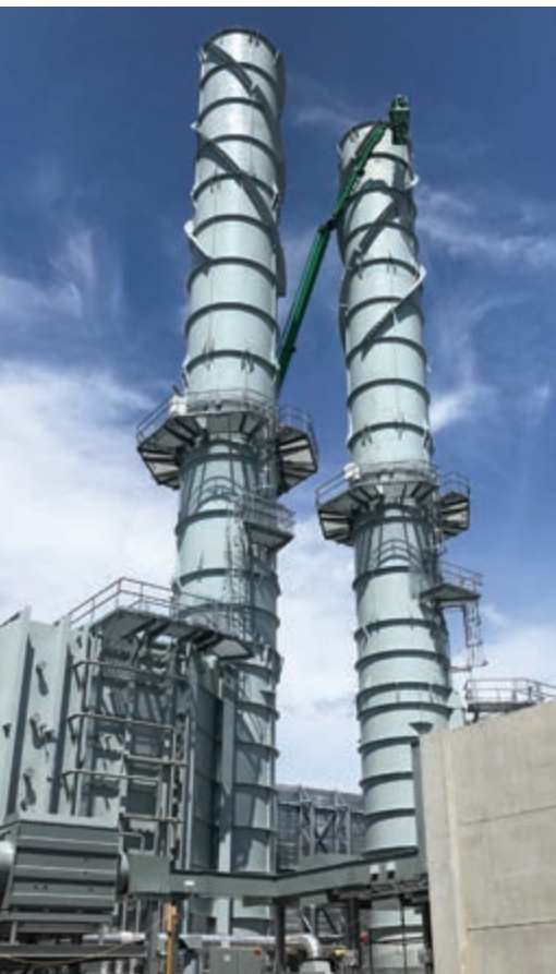
The coating on the finished stacks is designed to protect the steel at service temperatures of up to 500 F.
